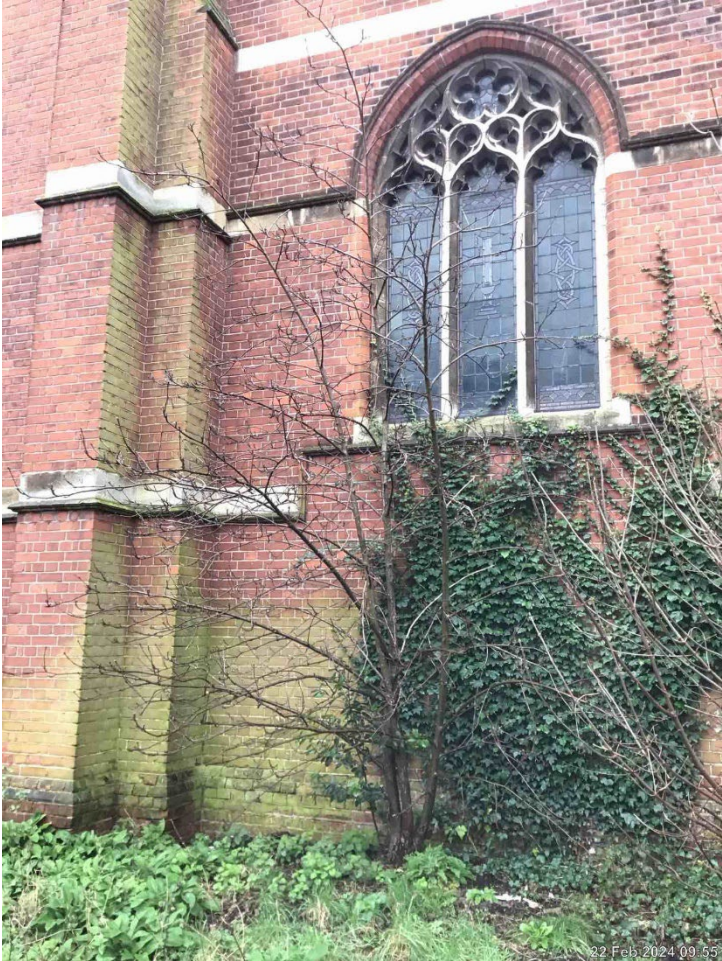
Images show tree in located in situ at the base of the wall of the church.
