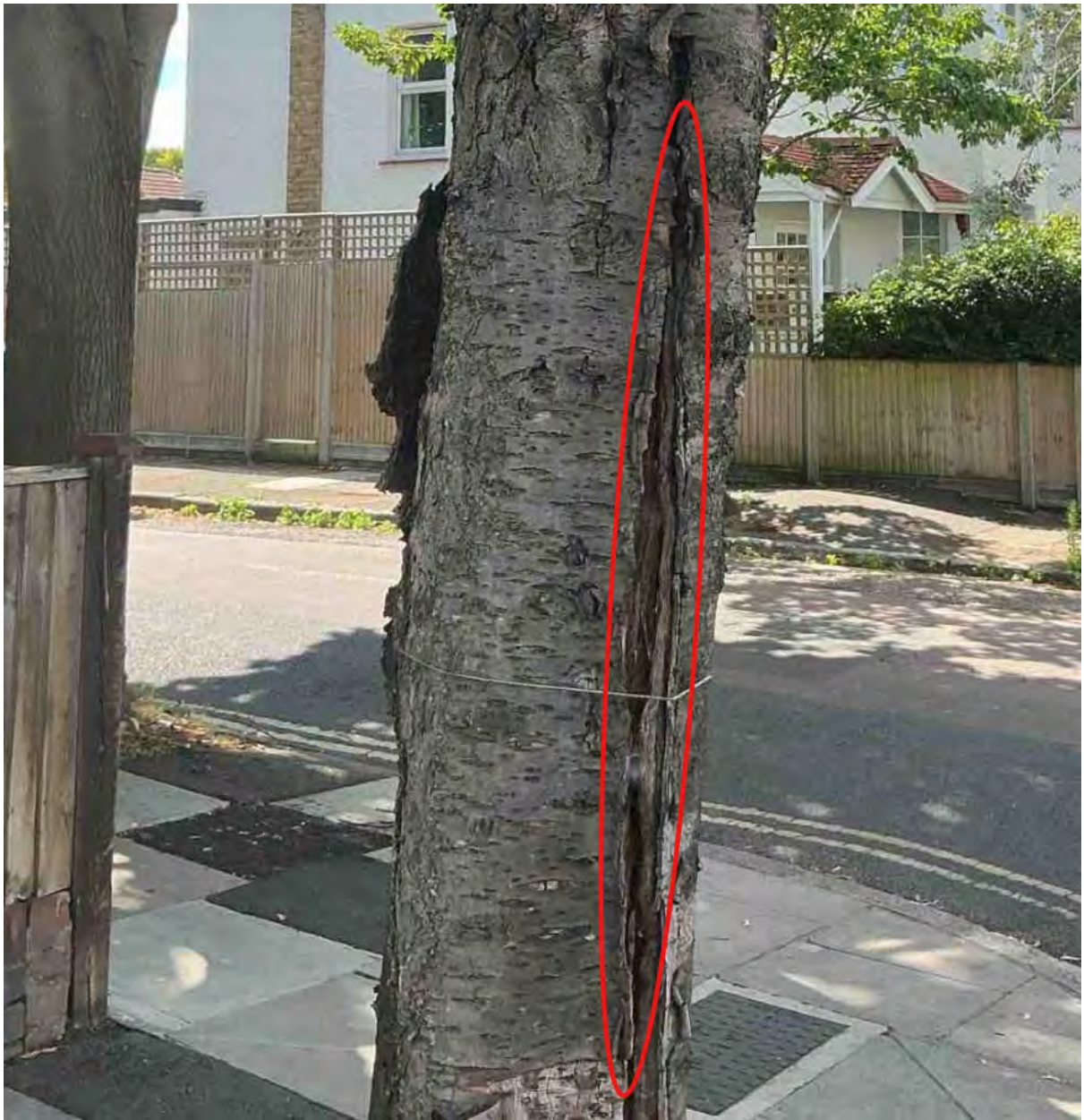
Image shows split in trunk circled
