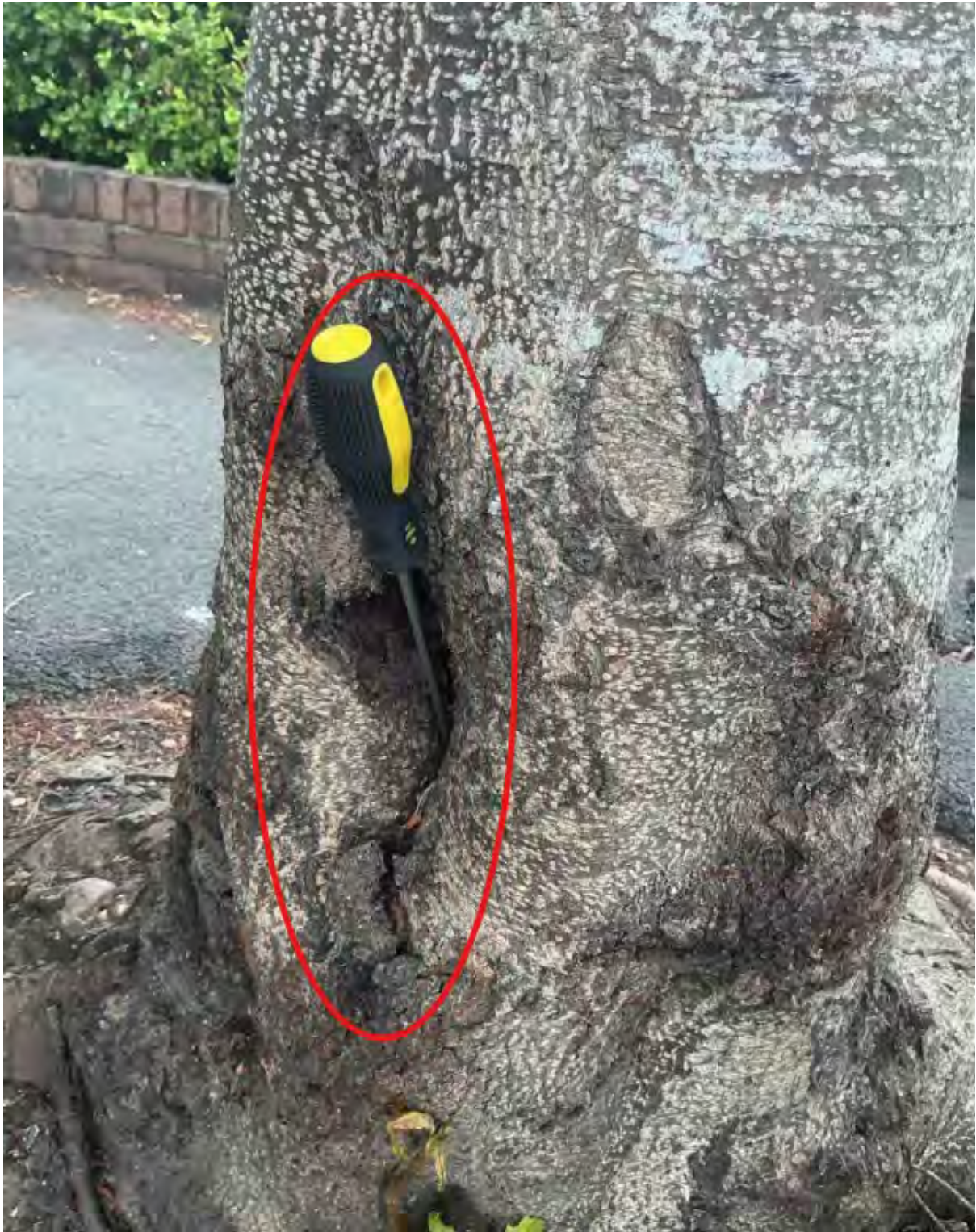
Image shows cavity with probe circled.
