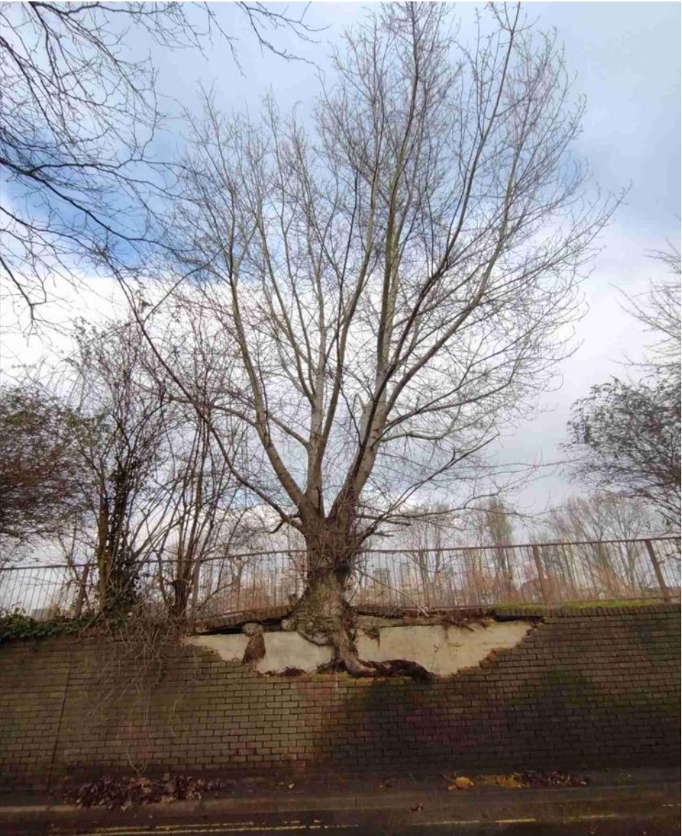
Image shows tree with damage to retaining wall and exposed flood defences
