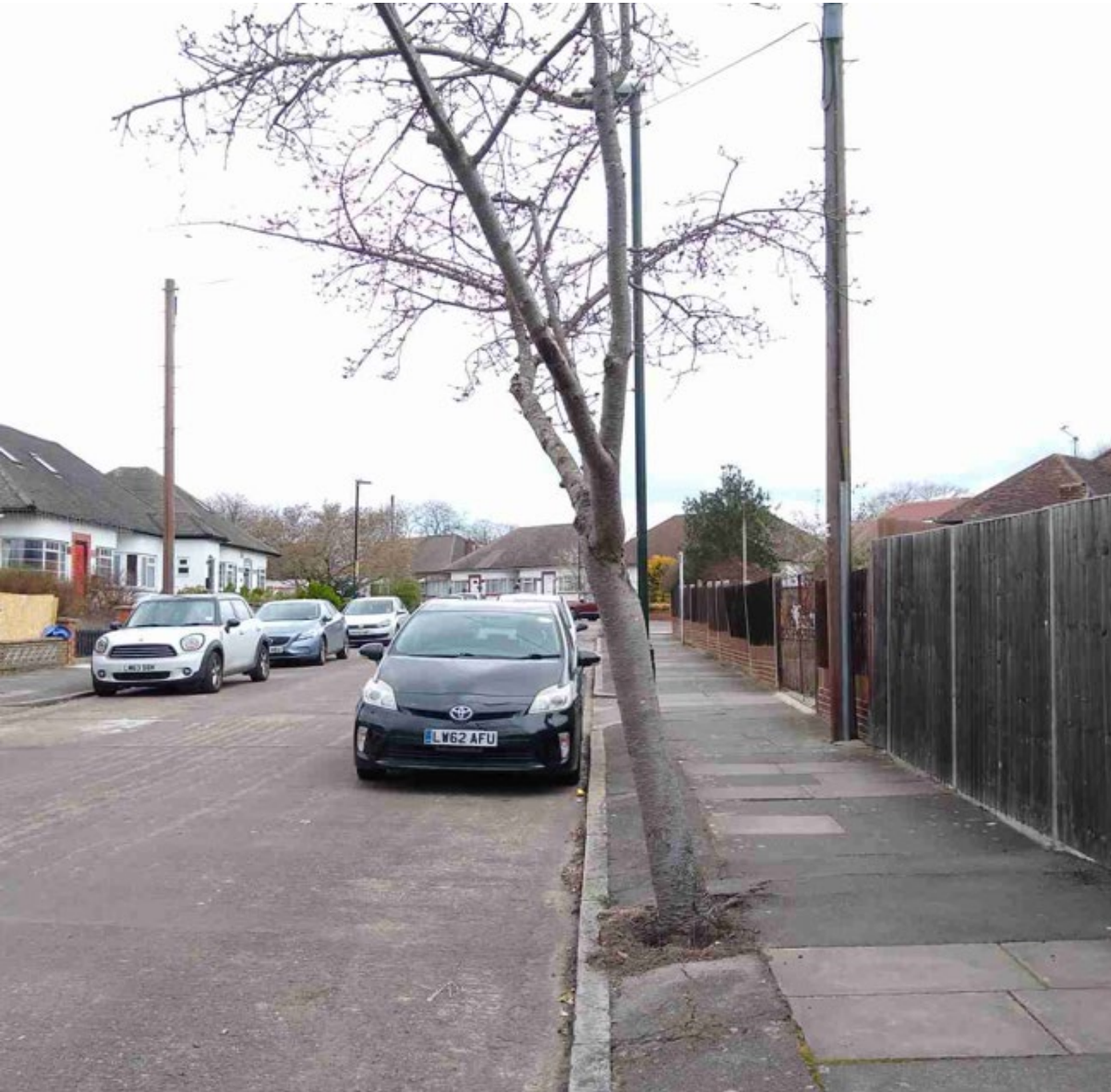
Image shows tree in street scene with signs of movement around base of trunk
