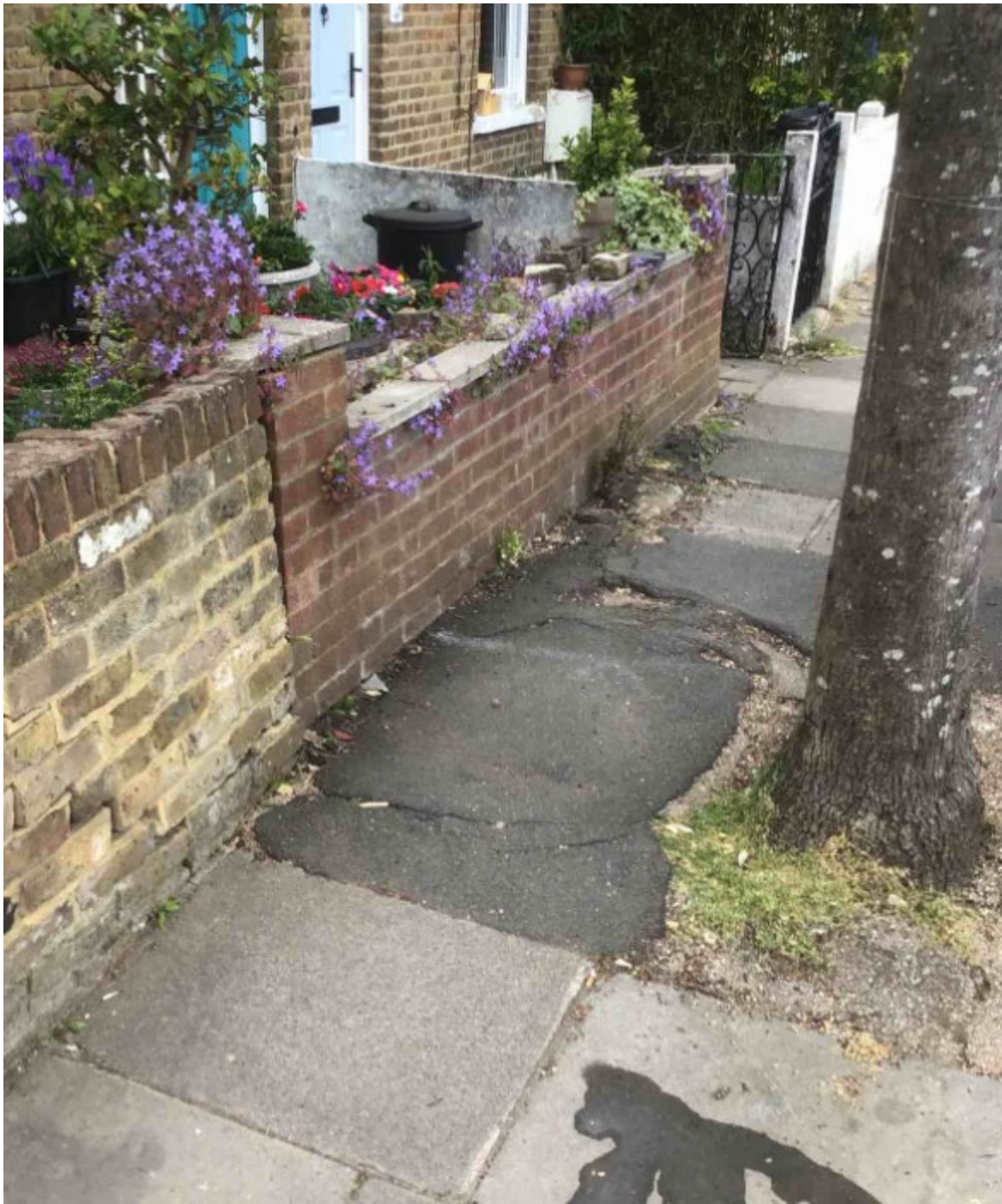
Image shows damaged narrow pavement due to tree
