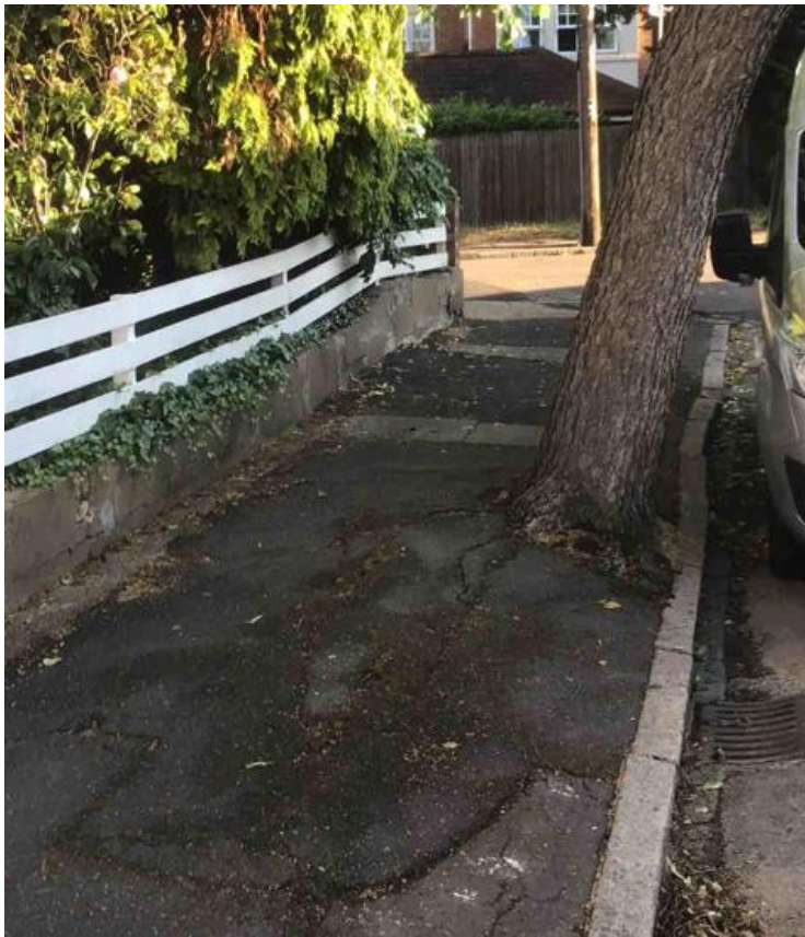
Images above shows pavement disruption with root heave caused by leaning stem
