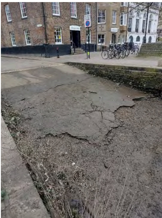
Figure 57 Water Lane slipway, with tarmac in poor condition
