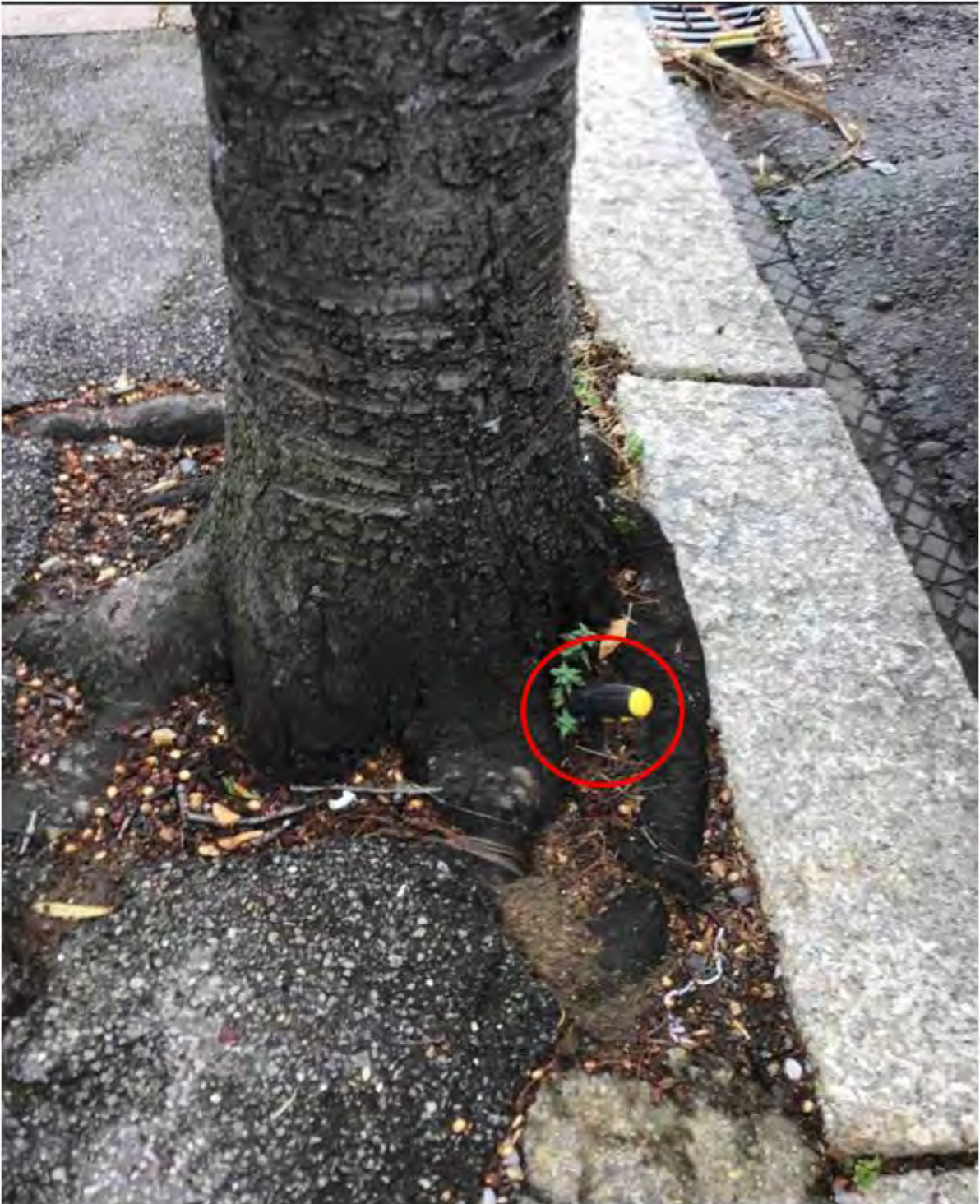
Image shows probe highlighting decay at base of stem circled.
