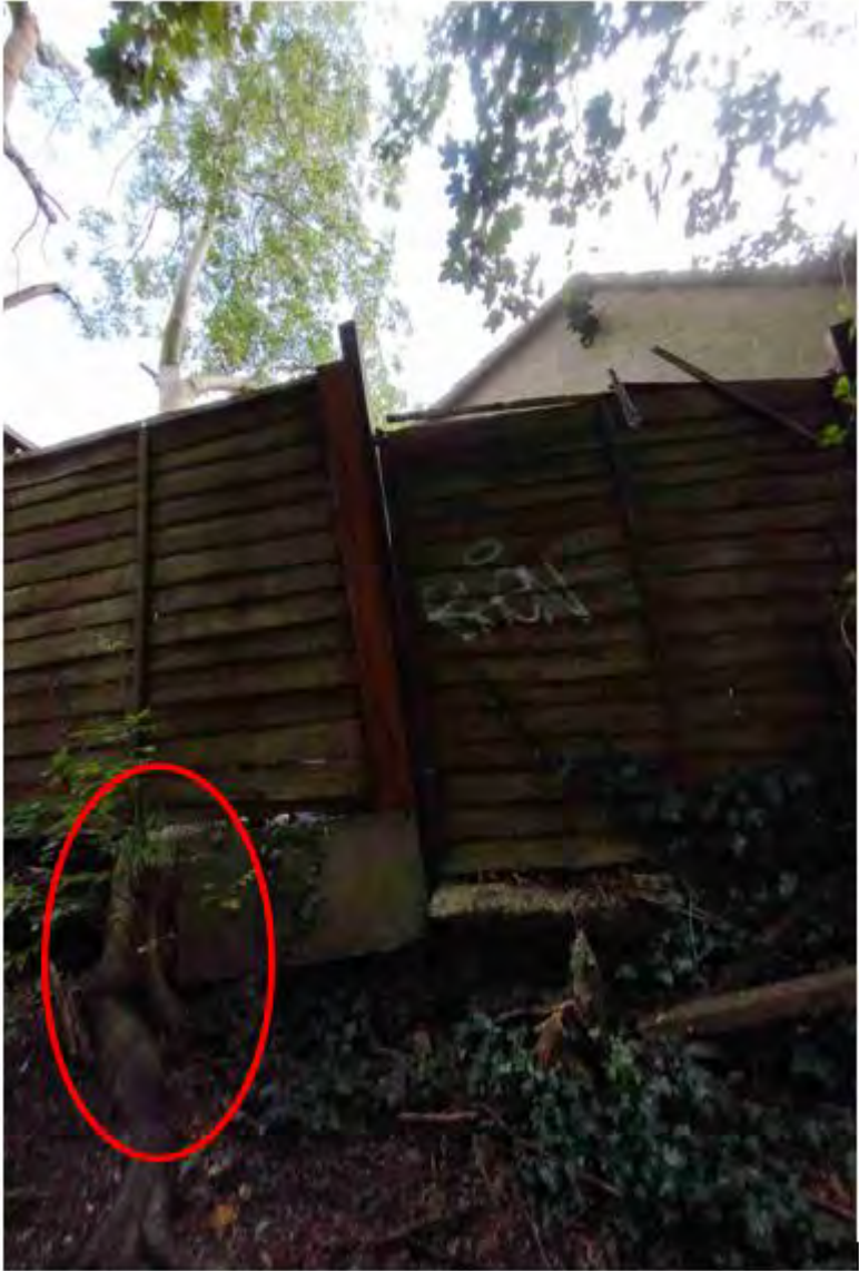
Images show tree in woodland context with base of stem damaging fence circled
