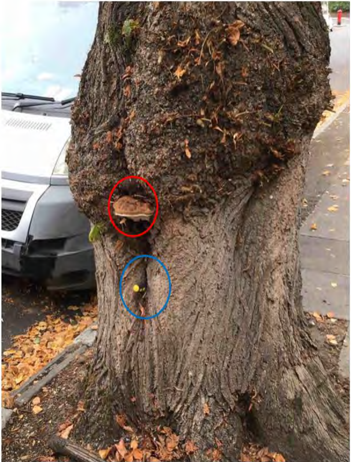
Image shows Ganoderma circle in red and probe circled in blue highlighting decay in stem.
