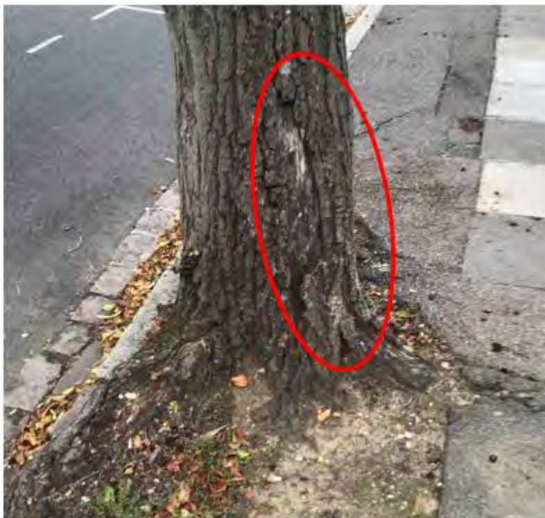
Image shows areas of delaminated bark circled in red at base of stem
