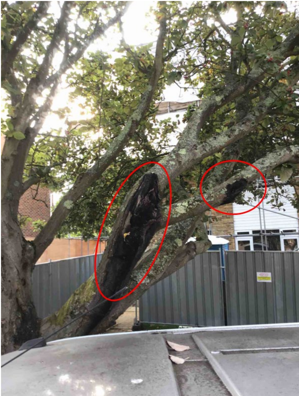
Image shows cavities from historic branch failure circled in red
