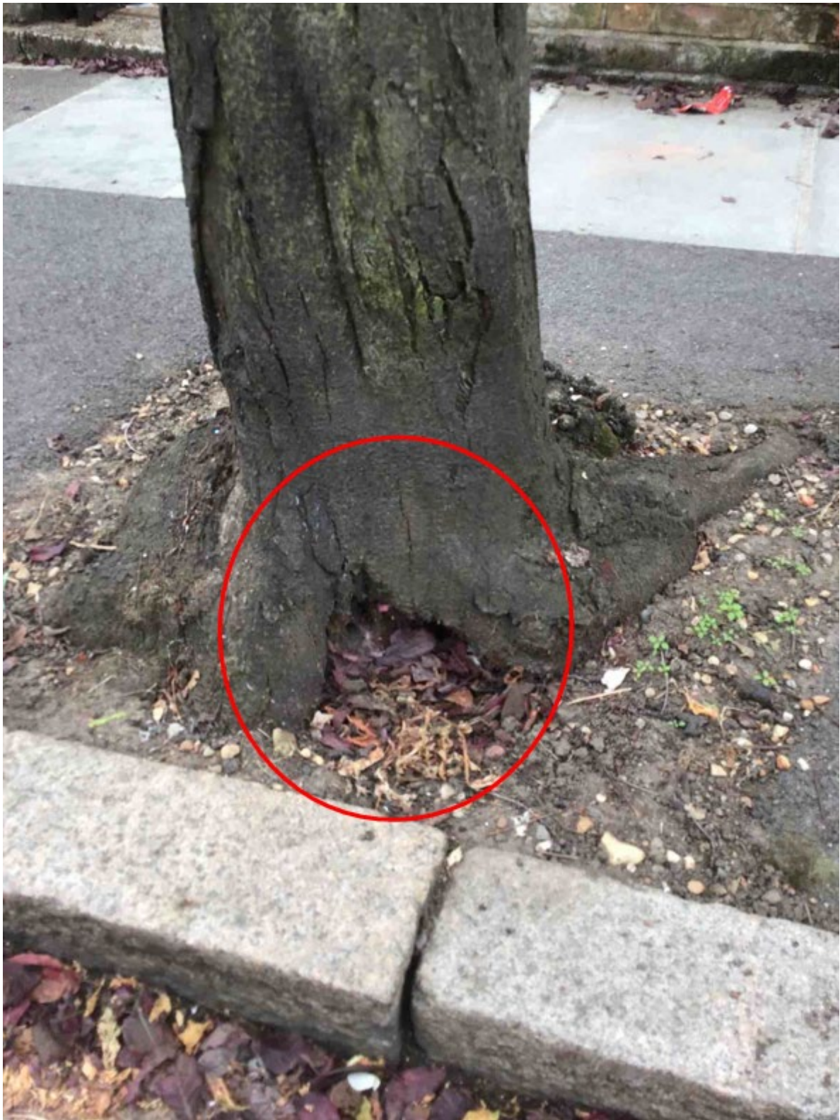
Image shows cavity at base of tree circled in red
