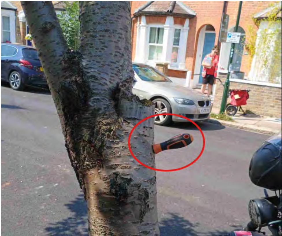
Image shows probe demonstrating decay on trunk circled.
