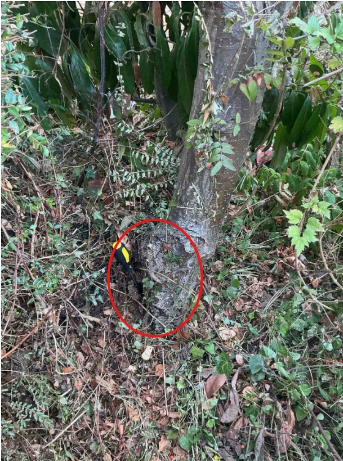
Images show cavity and probe circled.
