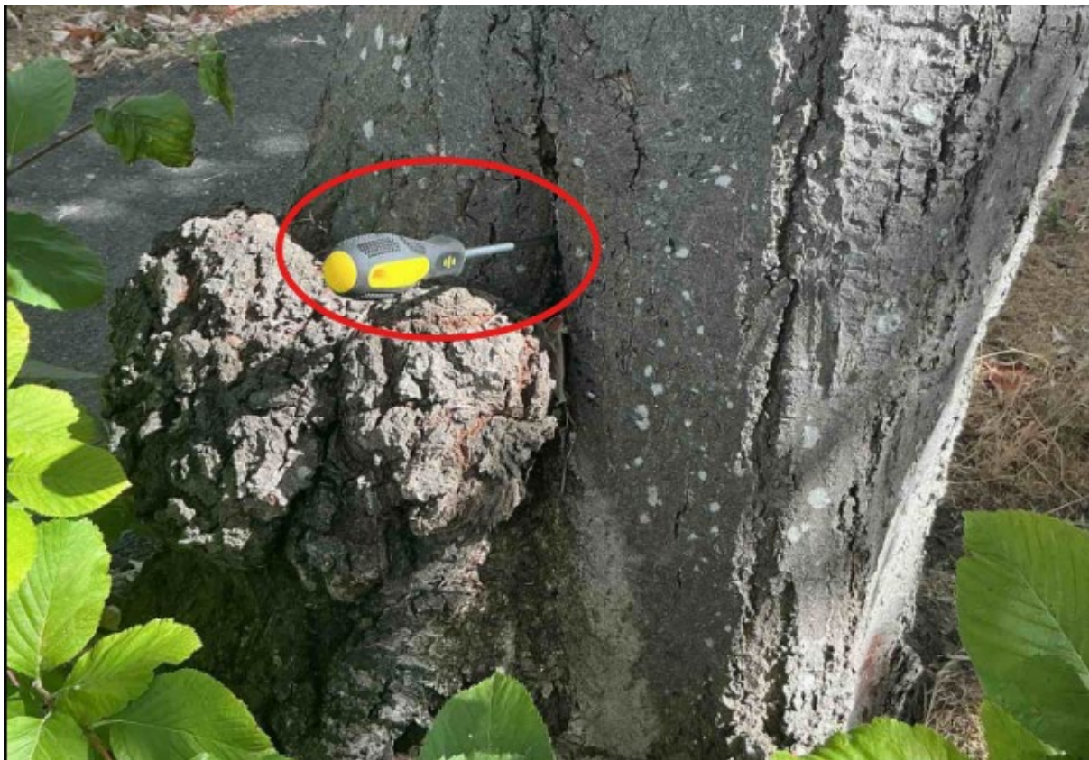
Image shows probe highlighting cavity at base of trunk.
