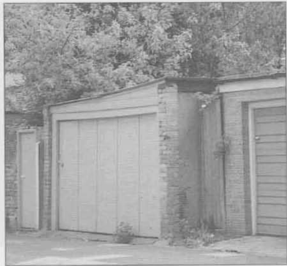
Unsightly garages facing onto Rosslyn Road
