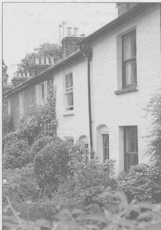
View along nos. 1-13 Park Cottages
