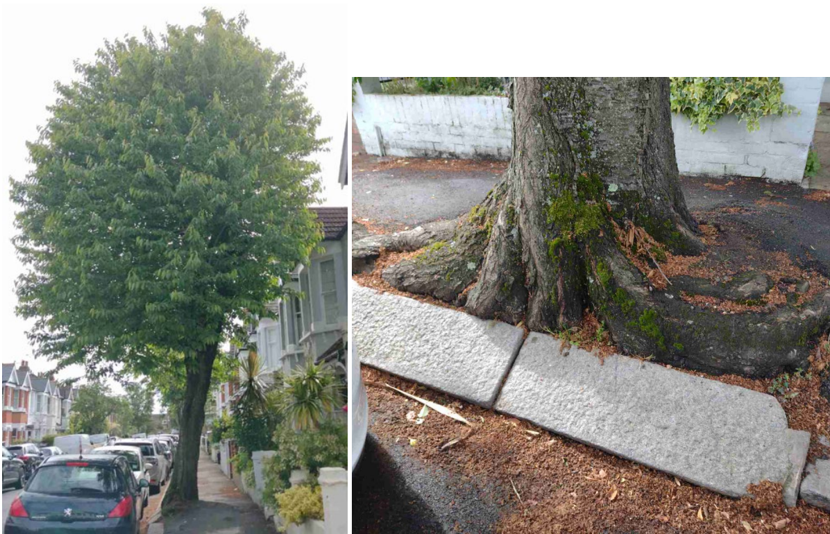
Left image shows tree in street scene, right image shows base and rooting disruption to pavement and kerb
