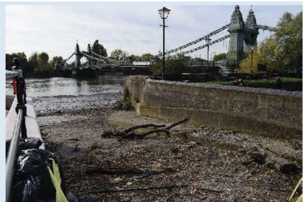
Looking southwest from the Queen Caroline Street flood gates. The corner river wall in centre frame will accommodate the northern abutment of the proposed temporary bridge with the bridge ramp extending rightwards along the river wall before meeting the ground at street level.
