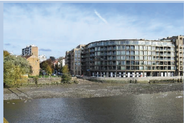
View from Hammersmith Bridge looking northeast to Hammersmith and the newly developed Riverside Studios that sit behind the landing area of the proposed temporary bridge centre left.
