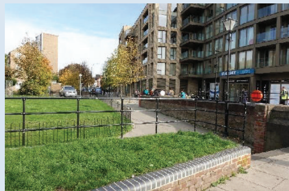
View northeast towards the southern end of Queen Caroline St from the north landing area of the proposed temporary bridge. The grassed area in the foreground will receive the bridge deck.
