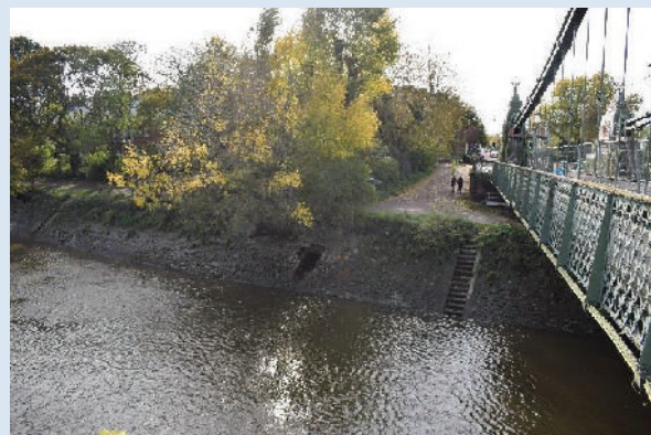
View from Hammersmith Bridge looking southwest to Barnes and the landing area and southern abutment of the proposed temporary bridge in centre frame.
