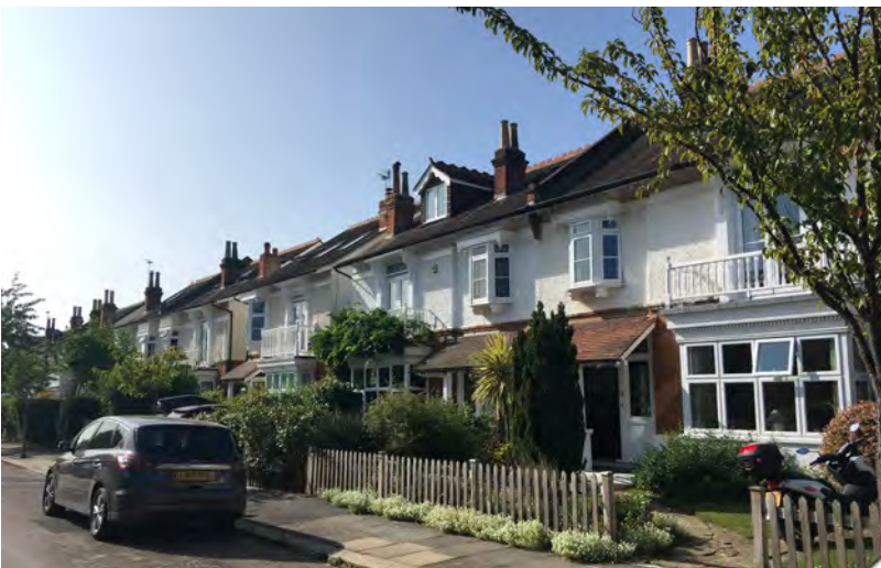
Row of houses with ground floor bays and timber balconies above, oriel windows and well greened front gardens.
