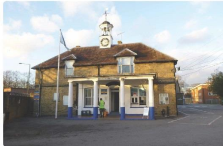
Main Guard Room
