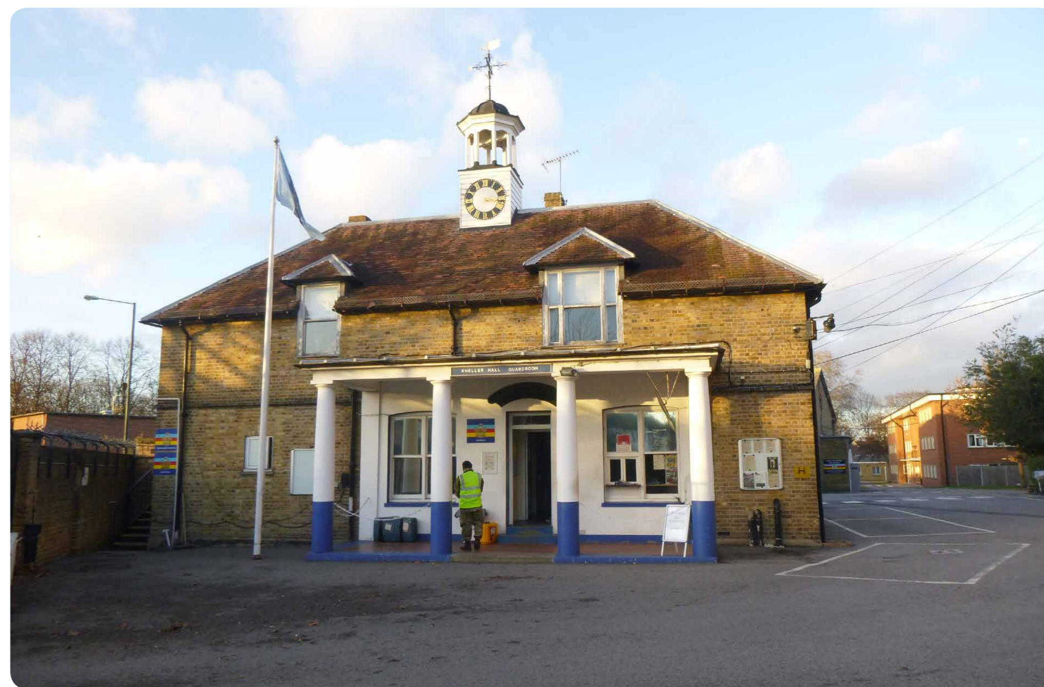
Main Guard Room
