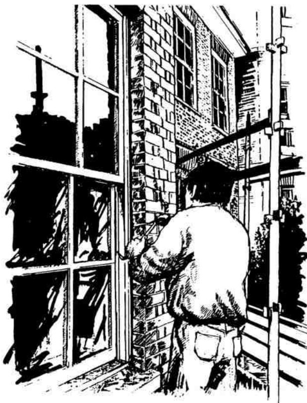
Tuck pointing being carried out to 'The Green' Hampton Court
