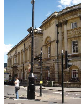
CCTV jumbo bases
