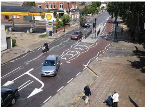
Excess road markings and lining
