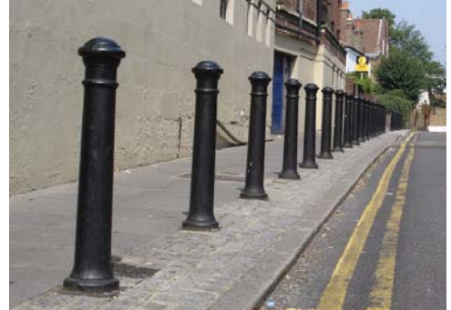
Overuse of bollards
