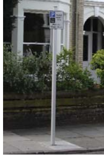
CPZ signage on galvanised posts
