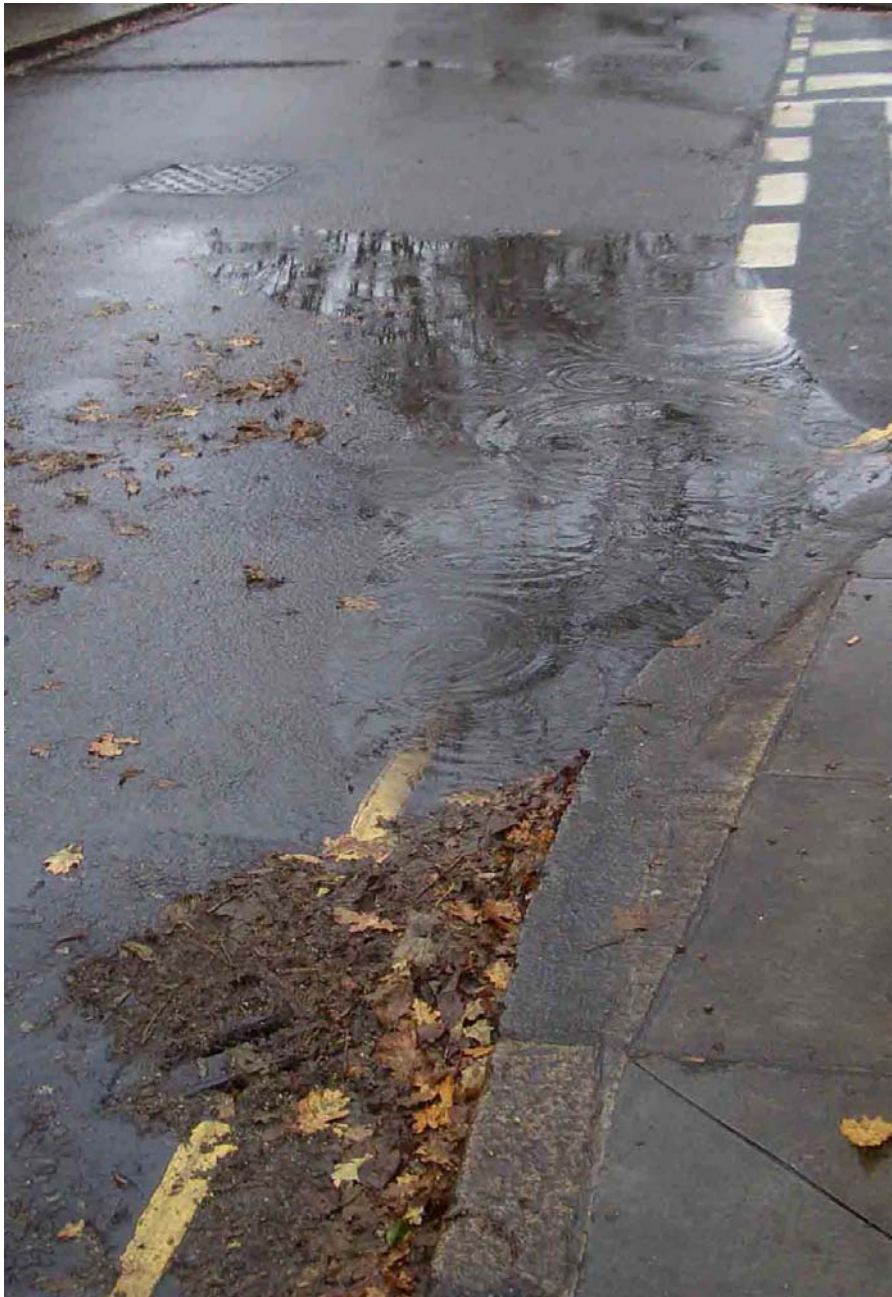
Surface water flooding at the junction of Amyand Park Road and Trafford Road caused by leaves partially blocking a drain, 25 December 2007.
