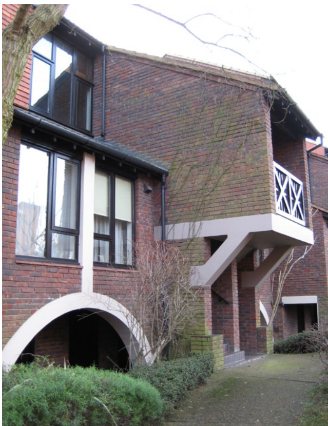
Exposed concrete supports add interest to the architecture of the building.
