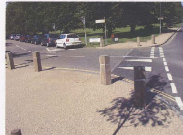
Timber bollards set in Heritage sealed gravel
