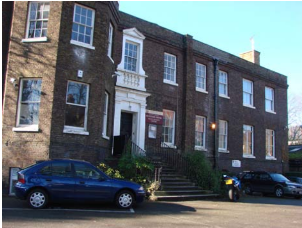
Front of Heatham House
