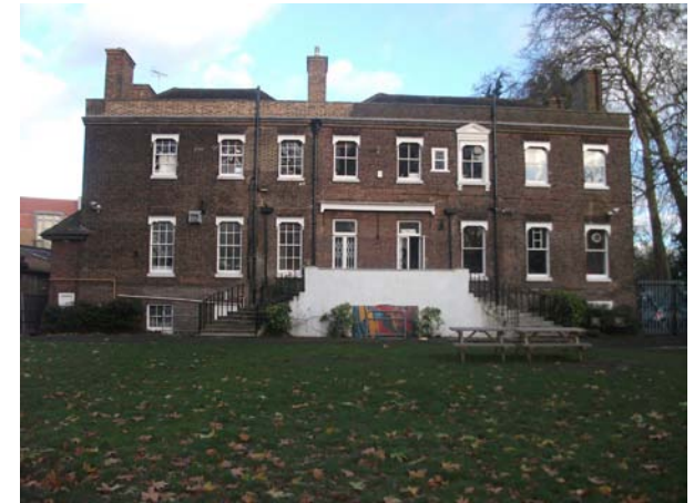
Rear of Heatham House
