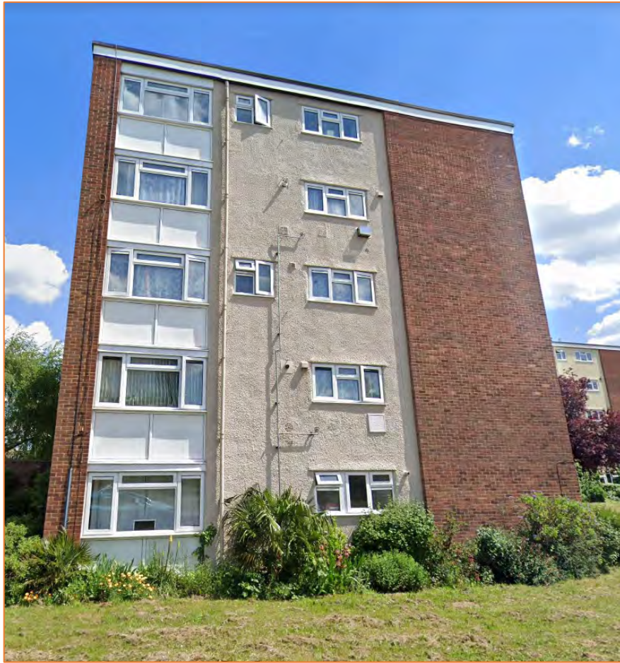
Figure 12: Existing Edwards House.
