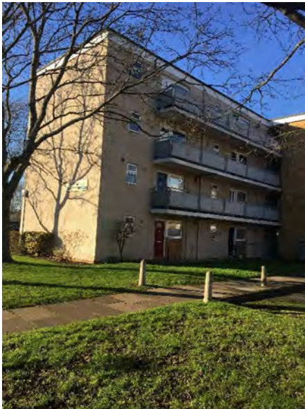
View of four storey block (Greig House).
