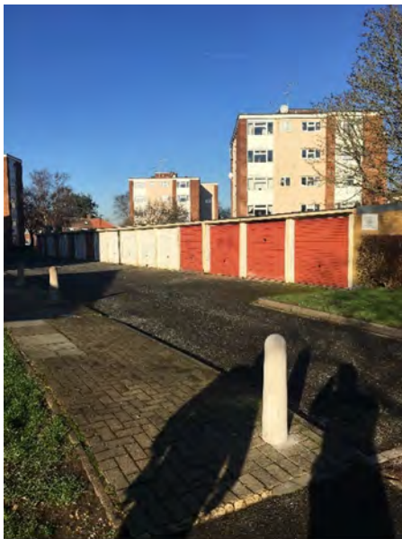
View of garages
