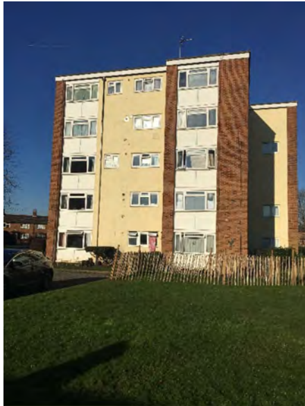
View of one of the five storey blocks of Ham Close
