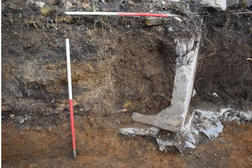
Plate 4: Modern concrete structure in Trench 2, looking northeast.
