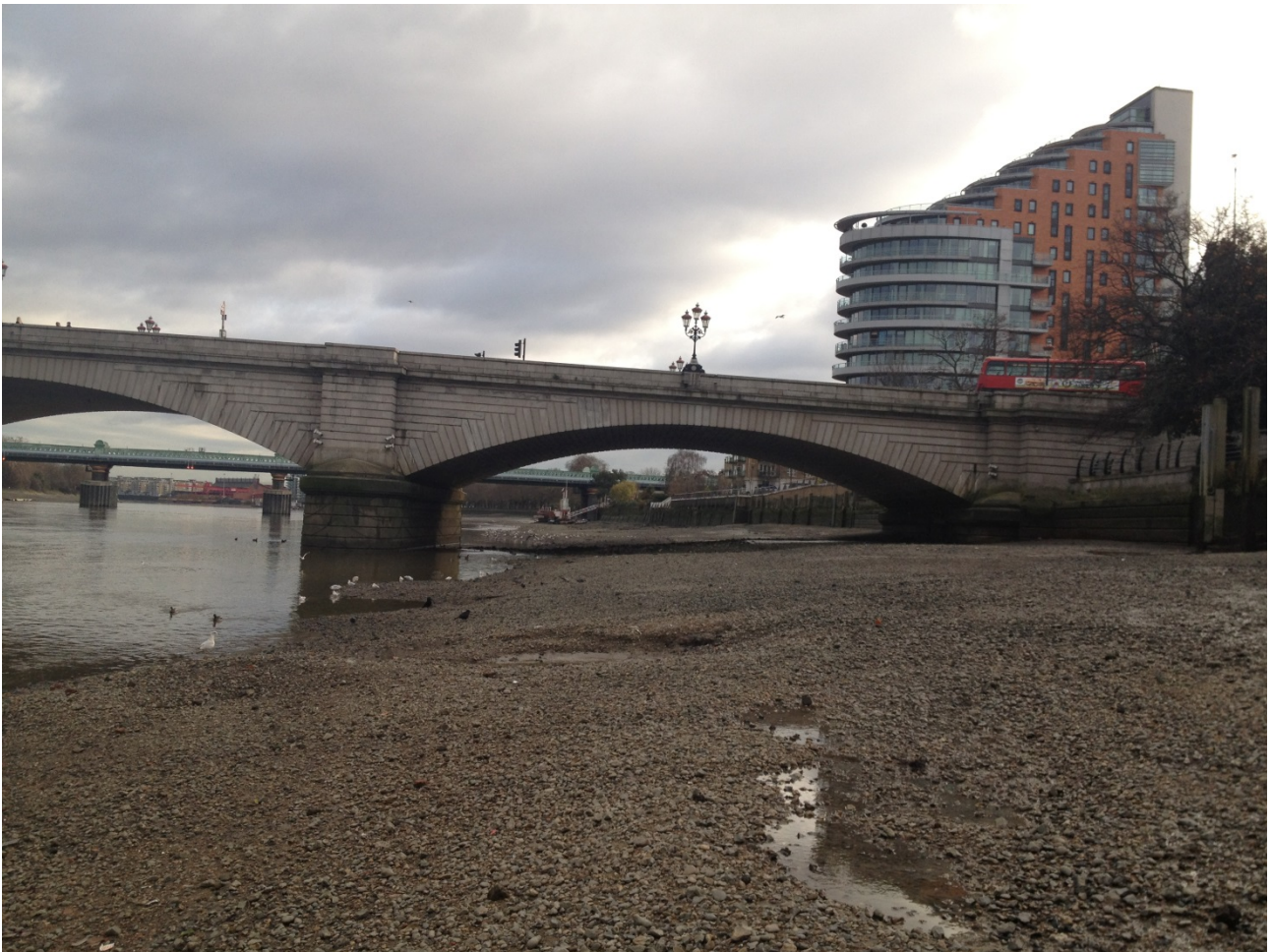
Photograph 4.1: South foreshore at Putney Bridge
