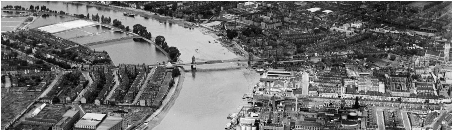
Fig. 13: Aerial view of Hammersmith and Castelnau, 1938
