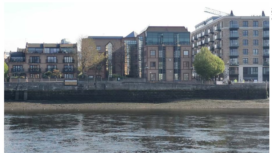
Fig. 36: Locally listed river wall, viewed from the southern Thames Path
