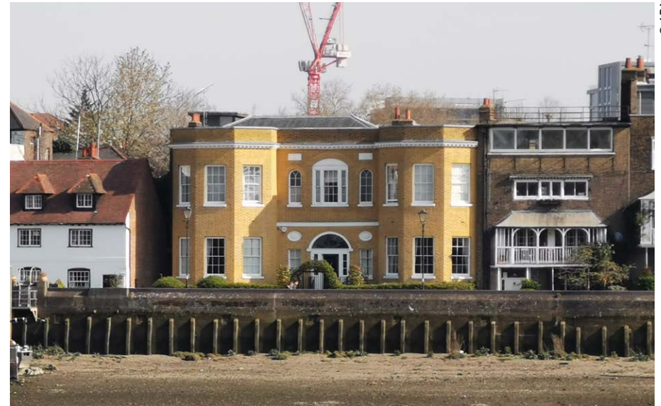
Fig. 22: No. 10 Lower Mall (Kent House)
