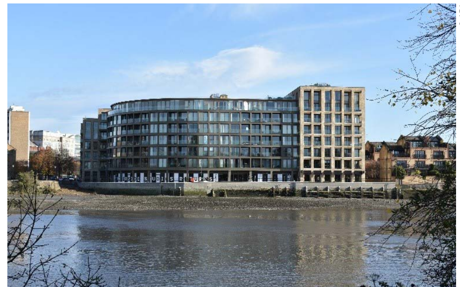
Fig. 15: Riverside Studios residential development, 2020
