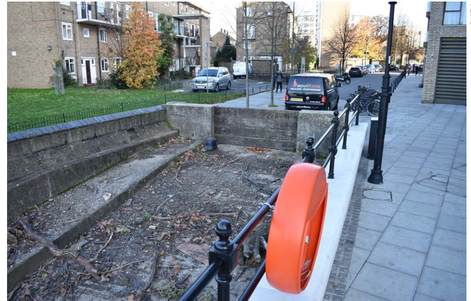
Fig. 35: Locally listed drawdock adjacent to the bridge
