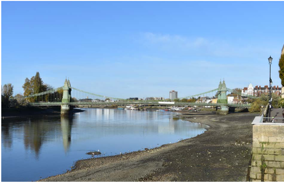
Fig. 54: View looking west towards Hammersmith Bridge from the northern Thames Path, 2020
