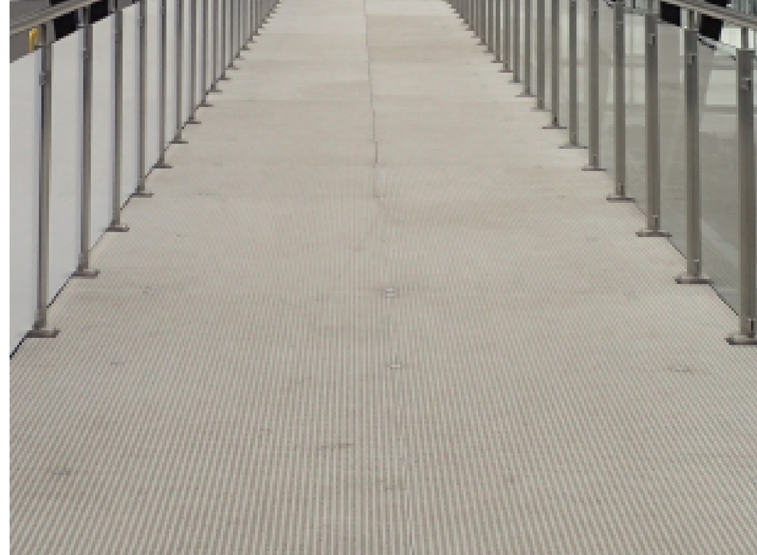
INDICATIVE LANDSIDE WALKWAY STEEL WALKWAY WITH RESIN BOUND DECKING AND GALVANISED STEEL HANDRAIL (SEE 2048-BRL-02-XX-DR-C-3140)
