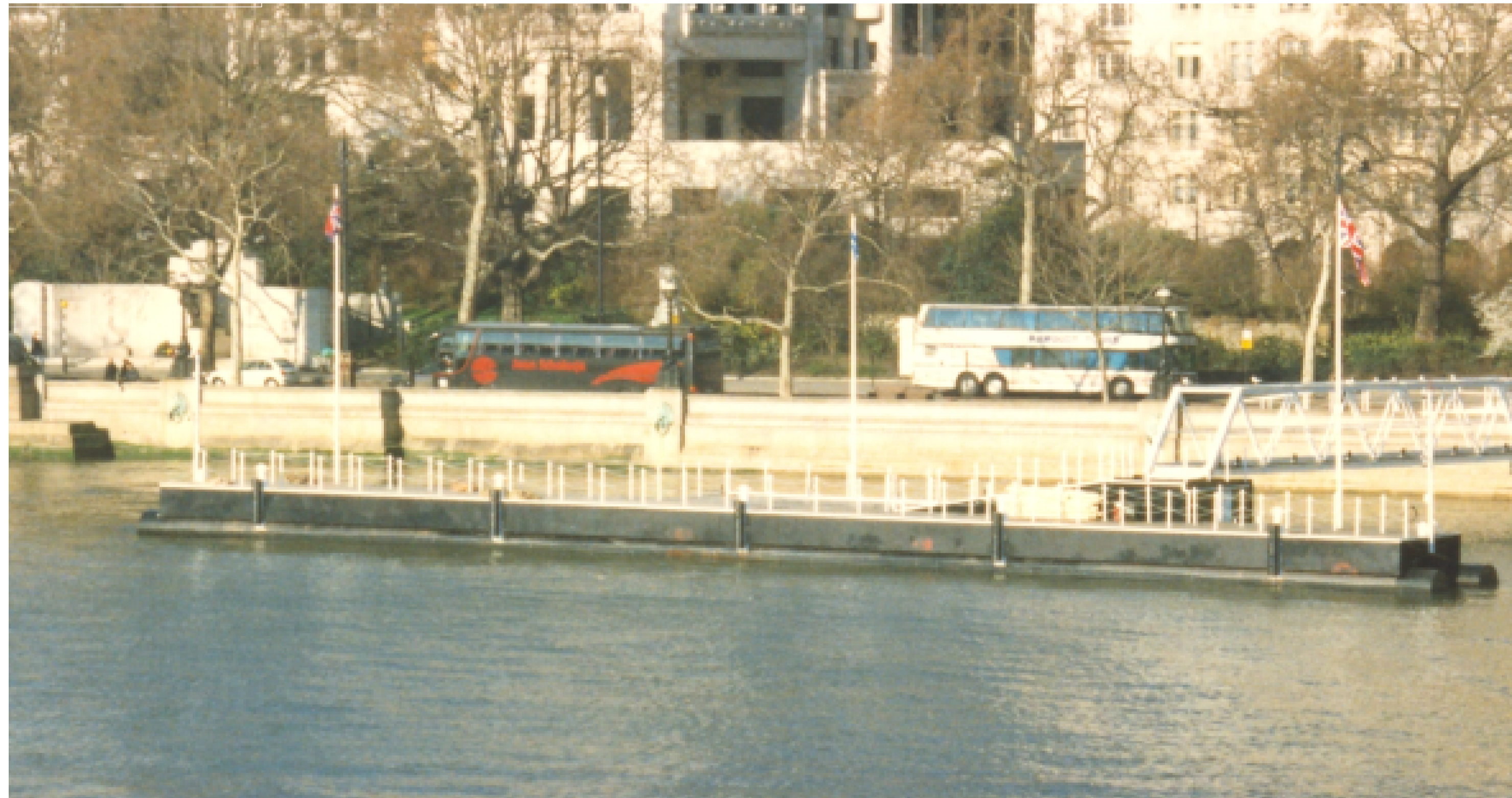
PONTOON PAINTED BLACK WITH RESIN BOUND DECKING (FOR FURTHER DETAILS ON SURFACING SEE 2048-BRL-02-XX-DR-C-3140)
