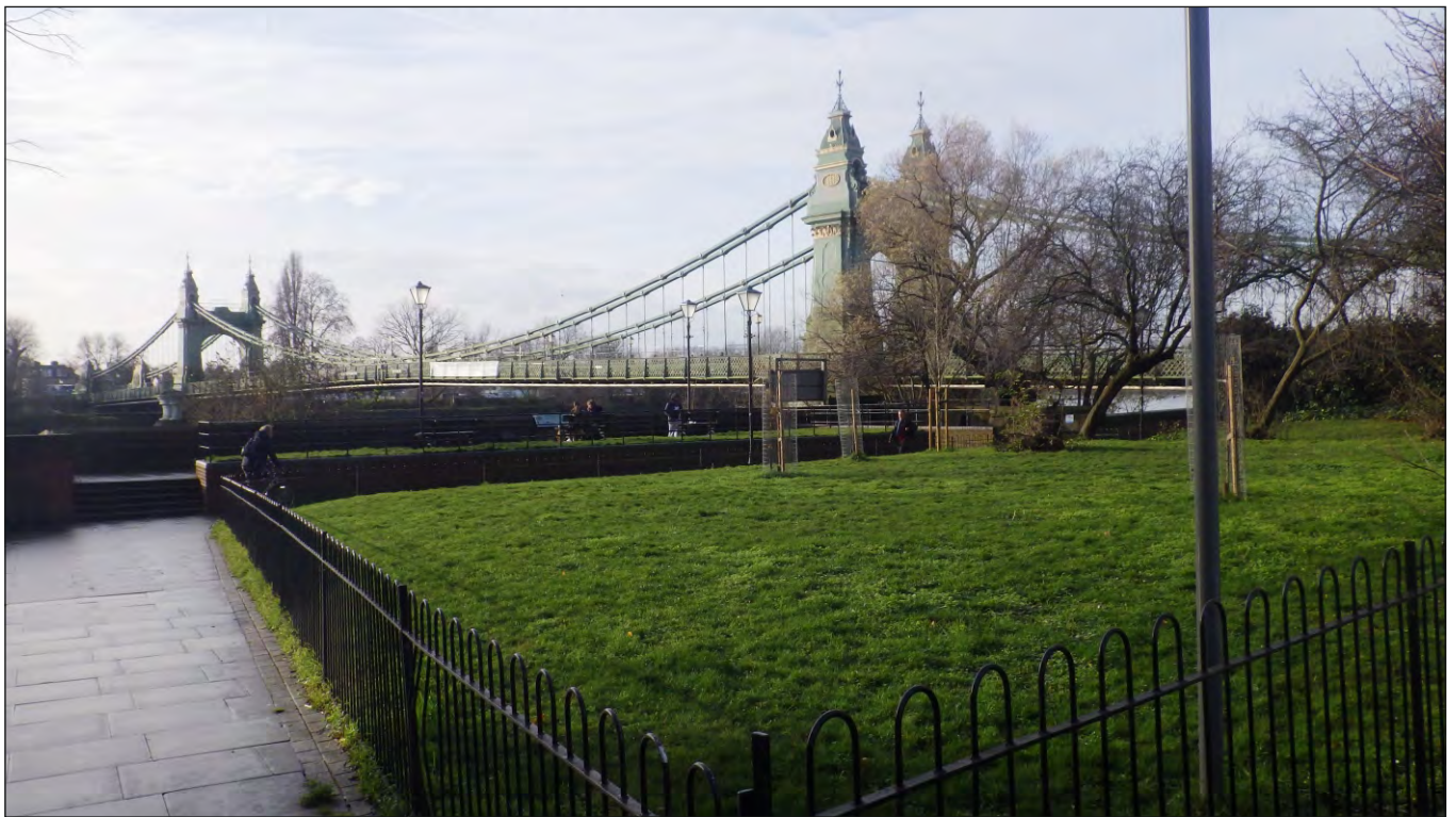
Plate 1: View of position of the northern abutment to temporary bridge (looking south) with Hammersmith Bridge in the background
