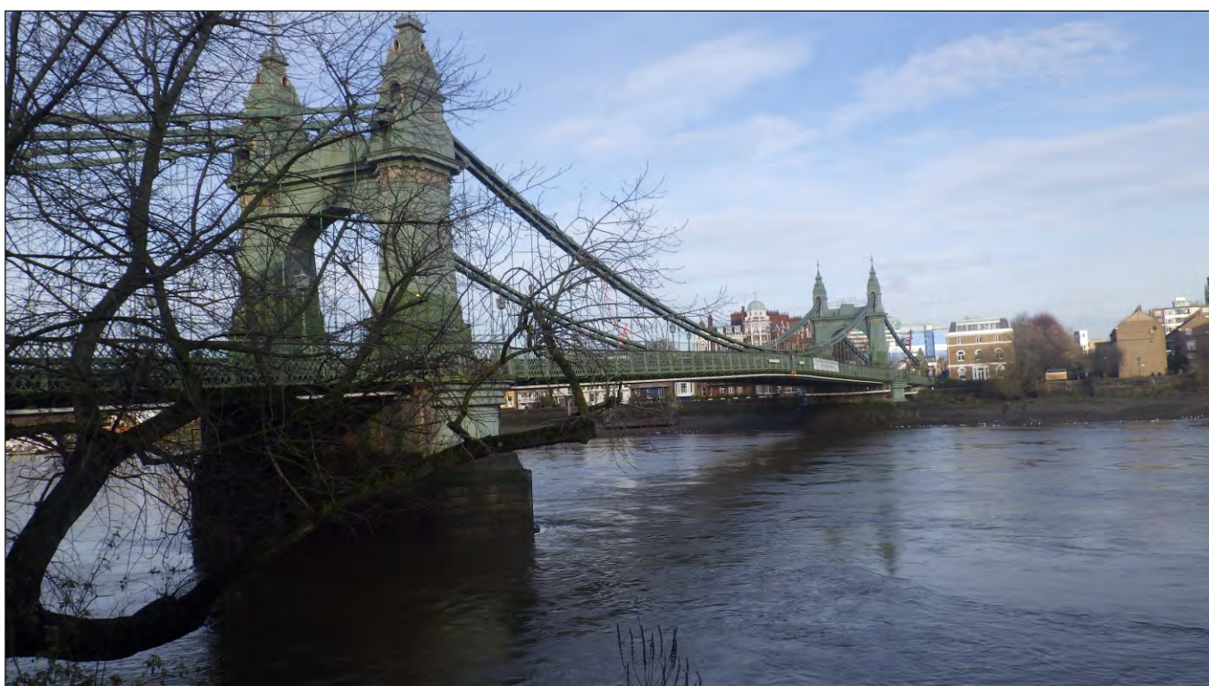
Plate 4: View of Hammersmith Bridge and the location of the proposed temporary bridge (looking north)
